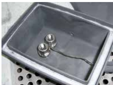
Brazing in a gas-supply box
